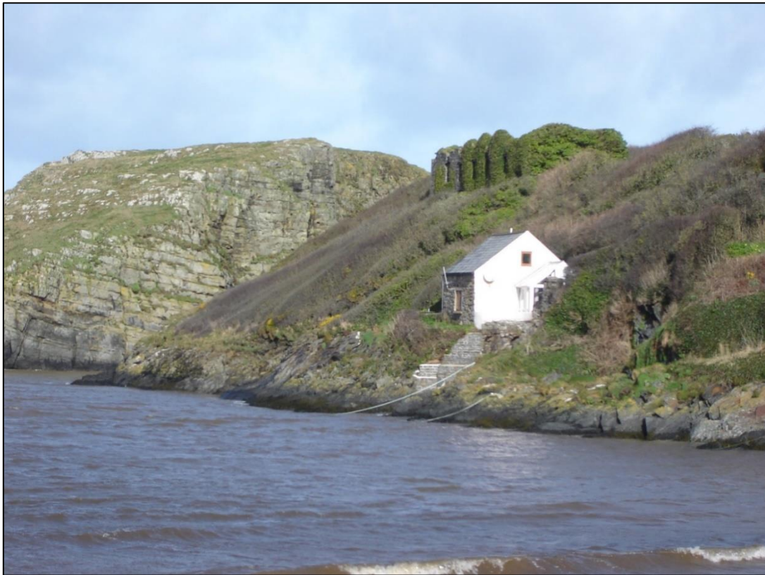
Doves Cottage / ex. Tap House Inn (with the Granary above).
