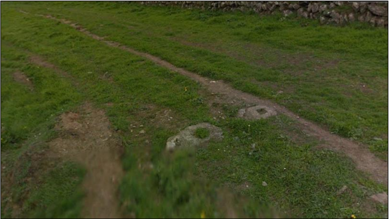
Fig. 73 The pair of Concrete Bases 2 on the cliff top.
