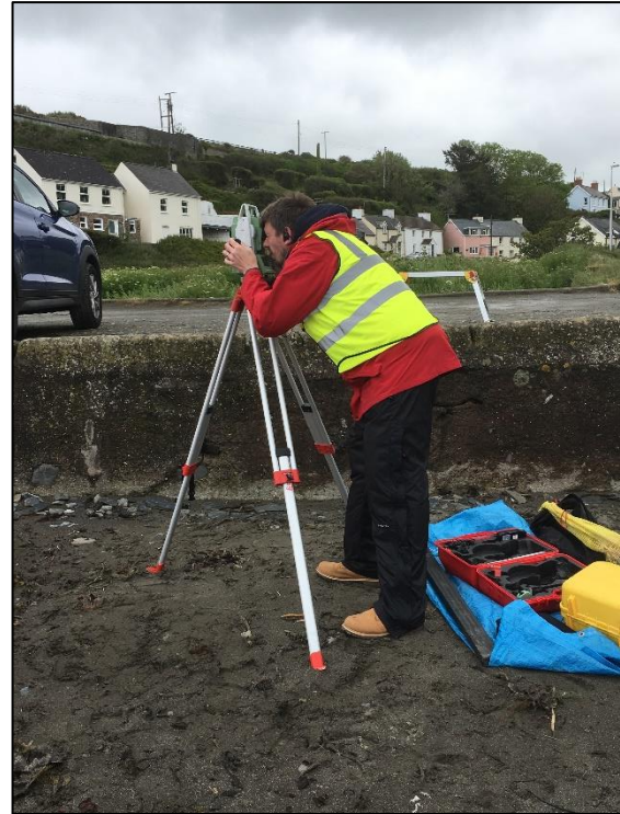
Fig. 38 Intertidal survey using the total station.
